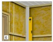
5. The first panel is cut and mounted at a distance of 10 mm from the floor and ceiling. 6. Use a leveler so the installation gets a right start.
