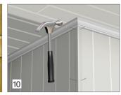
9. Use correction paint delivered in 20 ml to cover marks made by screws and nails. 10. For external and internal corners; use Huntonit's corner profile.
